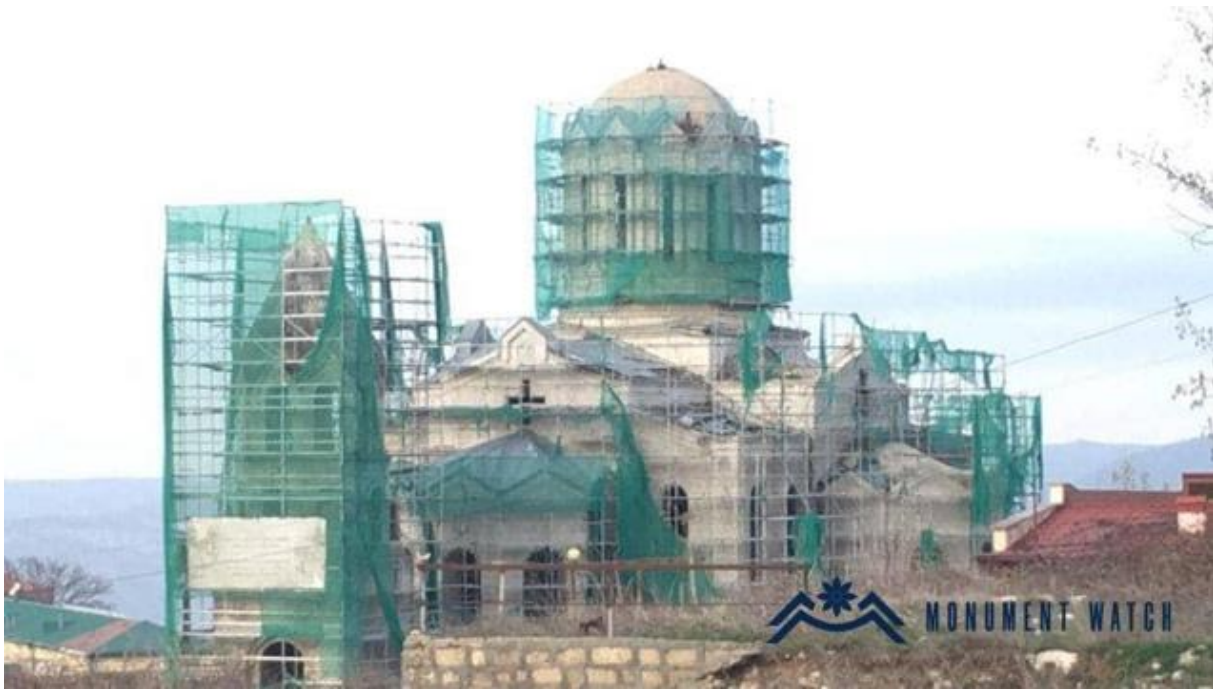
Figure 19: An Early Photograph of the Ongoing "Renovation" of Ghazanchetsots Cathedral. Monument Watch (2022).
